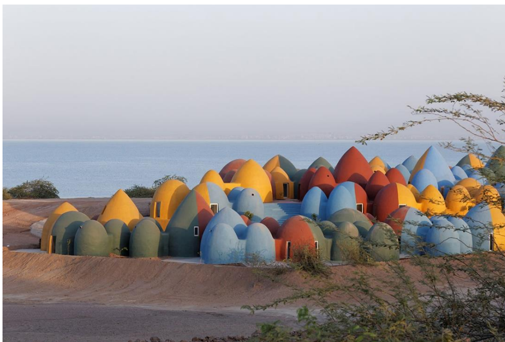
Architecture studio ZAV Architects has built a colourful-domed housing made of rammed earth and sand on Hormuz Island of Iran.
