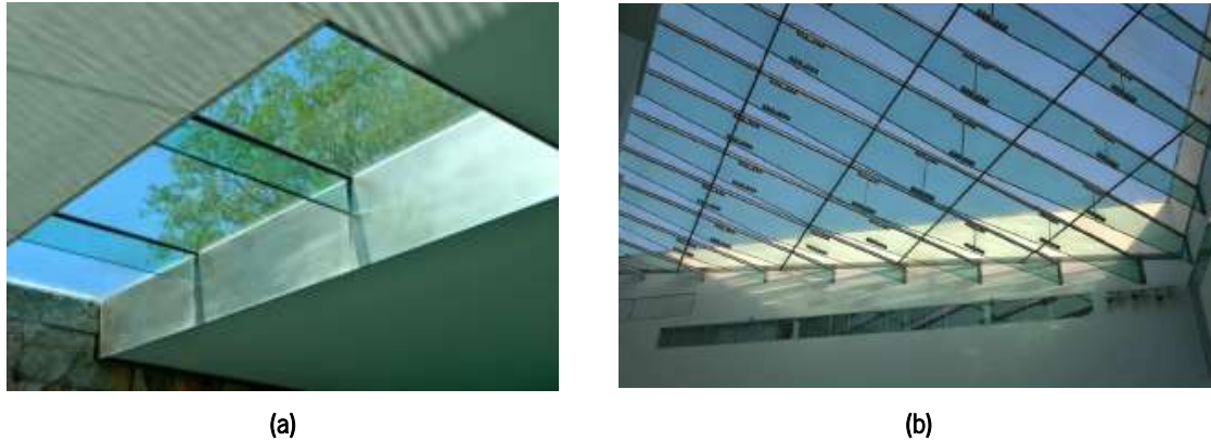
Figure 2.9: Types of glass beams: (a) continuous beams applied in a historic house in Ireland [54]; and (b) segmented-bolted beams designed by Arup for the Medical School building in Glasgow, UK [14].
