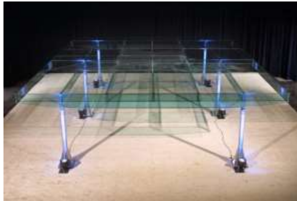
Figure 3.2: Fully transparent pavilion built at Delft University using steel-reinforced glass beams [31].
