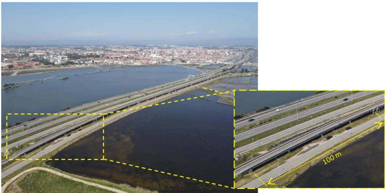
Figure 4. Extremity module of the west access viaduct of the Pirâmides bridge (Aveiro, Portugal).
