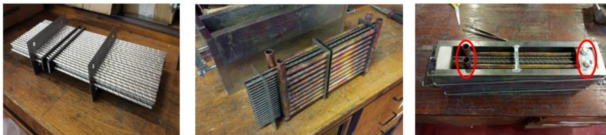
Figure 29 - (a) Corrugated pipes and (b) HPs arrangement before casting; (c) Corrugated Pipes and HPs inside de moulding box ready for casting.
