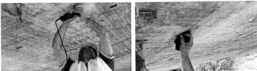
Figure 2. Surface blasting and cleaning
