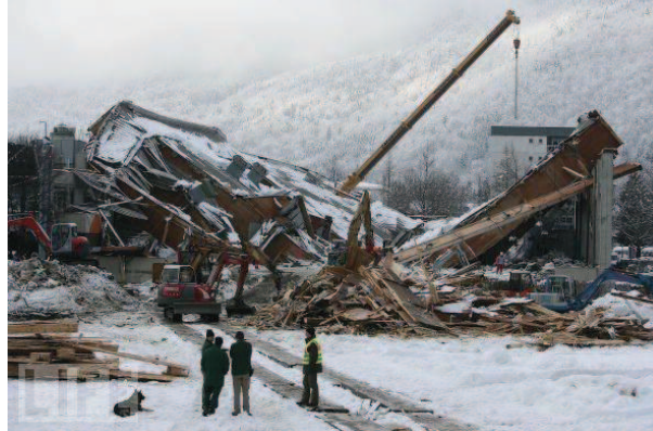
Figure 3 – Bad Reichenhall ice-arena collapse
