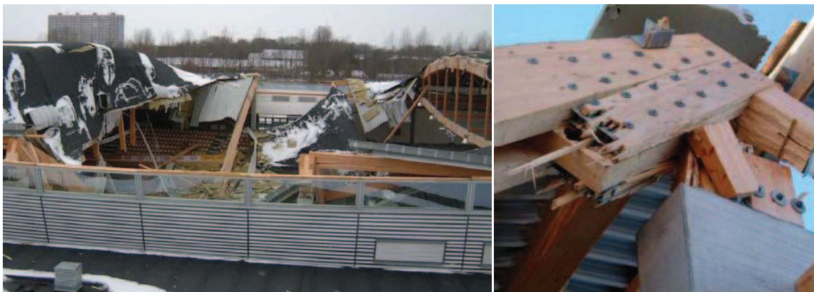
a) An intact truss is seen to the right
