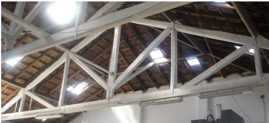
Figure 1 – Queen post truss analyzed
