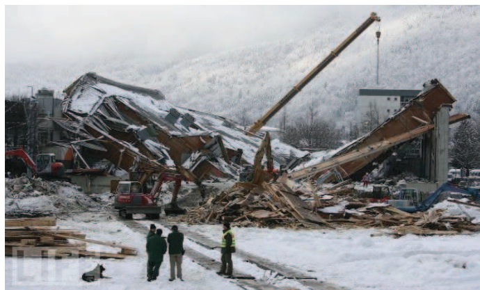
Figure 18. Bad Reichenhall ice-arena collapse
