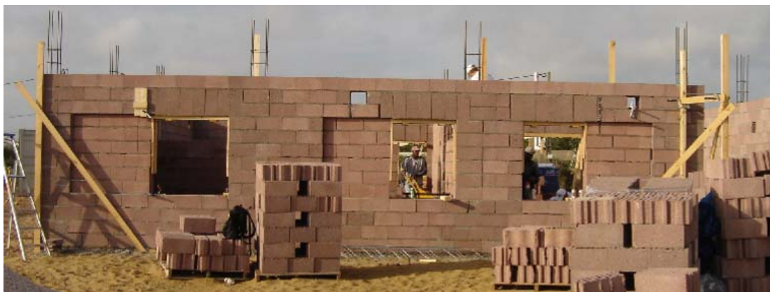
Figure 13 : Example of modern confined masonry under construction.
