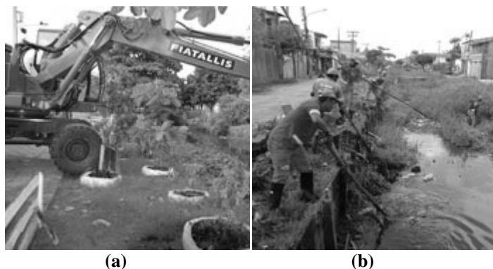
Fig. 6 – Cleaning and unclogging of Belém-PA channels. (a) dredging, (b) manual cleanup. Source (SESAN, 2011)
