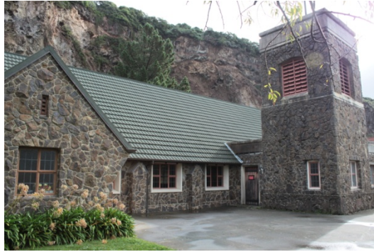
Figure 14 – Example of an undamaged church classified red due to instability of the slope shown in the background (All Saints, stone, Sumner).
