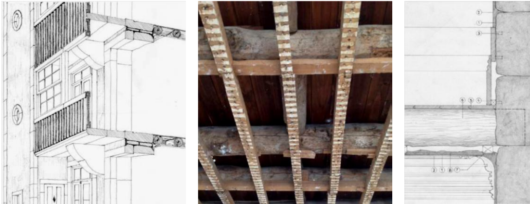
Figure 3. 17- Schematic axonometric representation of a typical 19th century Porto House's façade, Figure 3. 18-Picture of a typical wooden beam pavement, Figure 3. 19- Connection between wooden beams and the lateral granite wall
