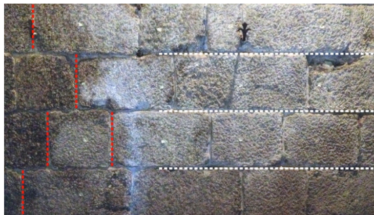
Figure 7. 6- Geometric characteristics of the inspected wall
