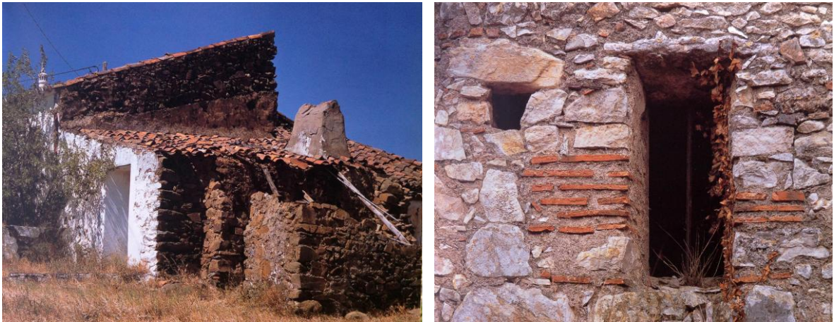
Figure 3. 4- Southern house built in limestone and earth, Figure 3. 5- Southern house built in limestone and brick. (From: Casella, 2003)
