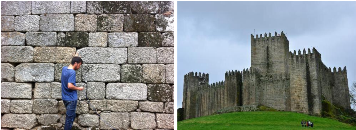
Figure 3. 32- Masonry of Guimarães castle, Figure 3. 33- Guimarães castle current condition
