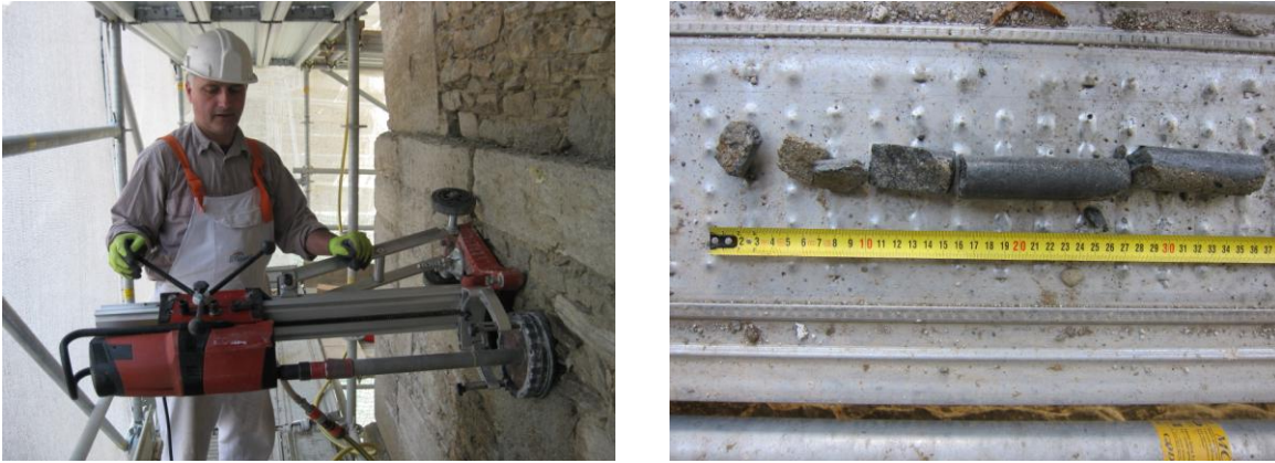
Figure 2. 15- The coring process, Figure 2. 16- Drilled core from a masonry wall
