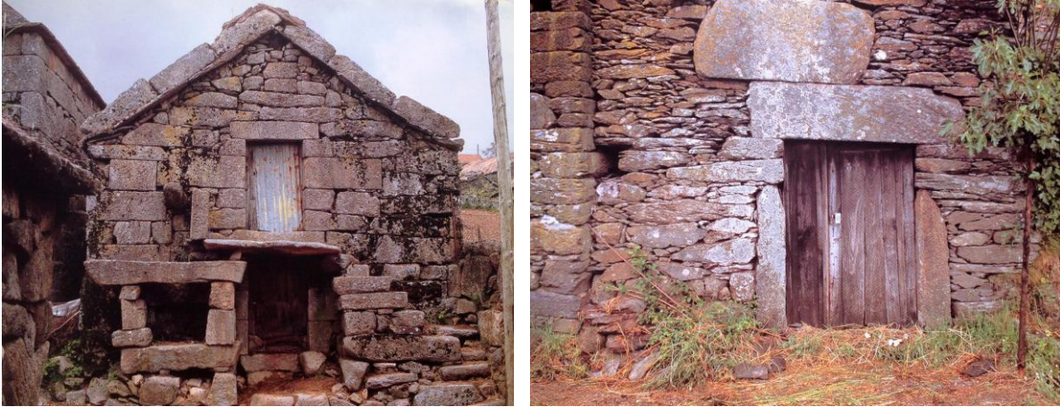
Figure 3. 2- Northern house built in granite. Figure 3. 3- Northern house built in mixed schist and granite (From: Casella, 2003)
