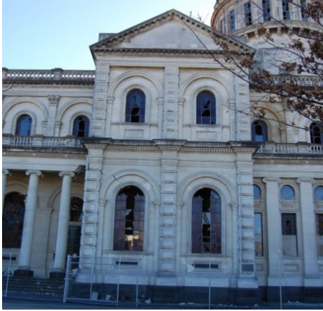
Figure 25 – South transept facade.
