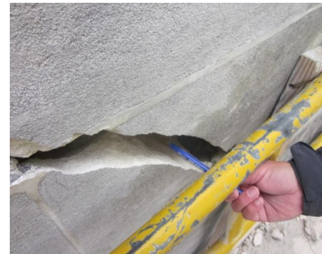
Figure 29 – Lateral displacements of the main dome drum or rotunda.
