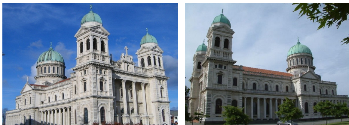
a) b) Figure 17 – Cathedral of the Blessed Sacramento: (a) North and West façades; (b) South façade.
