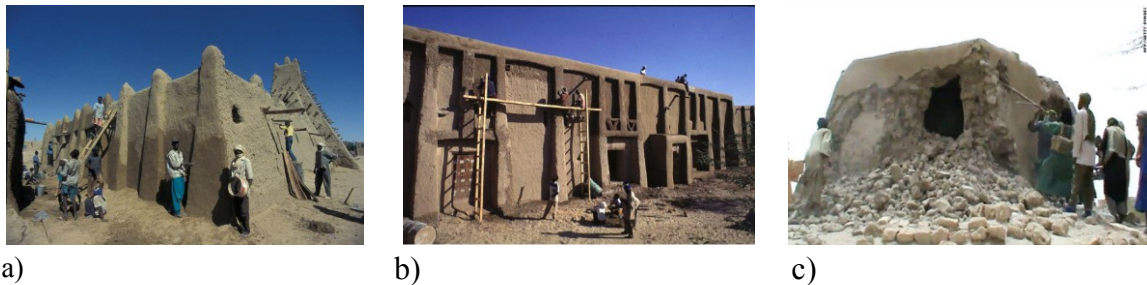
Figure 6 – Temples in Mali: (a) Restoration of Sankore mosque [25]; (b) Restoration of Djingareberre mosque [25]; (c) Destruction of a muslim saint tomb (Source: www.cnn.com ).
