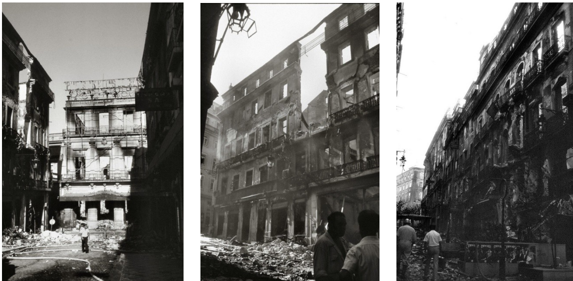
Figure 9 – Destruction of Chiado buildings by the fire in 1988 (Courtesy of Lebreiro Henriques : http://www.flickr.com/photos/lebreirohenriques/ ).
