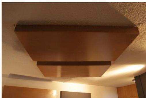
Figura 20 – Membrana ressonante [lemovacustica.com].
