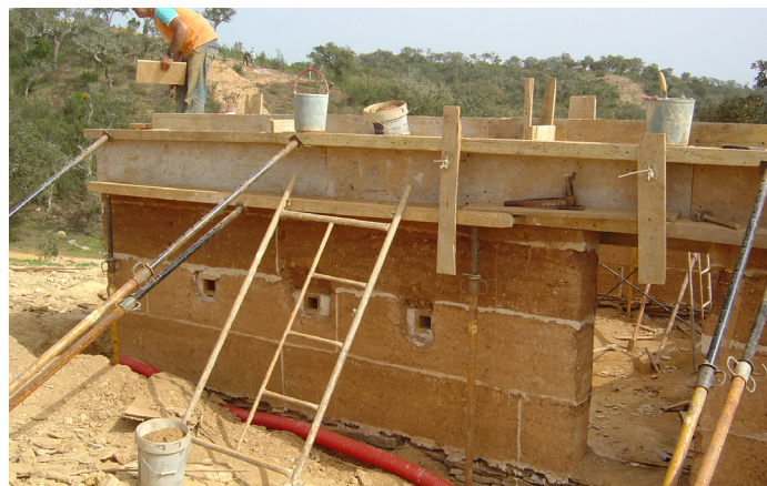
Figure 1: New rammed earth construction in Odemira (Portugal).
