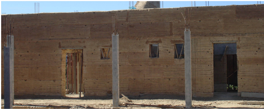
Figure 1. Rammed earth house being built in Odemira, Portugal.
