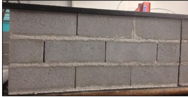
Figure 7.5. Masonry wall specimen without any reinforcement.
