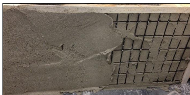
Figure 7.7. Structure reinforcement at one side of the masonry wall specimen.
