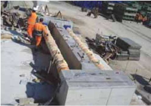
Figure 1: RG8 test – large dimension beam with restrained shrinkage [1]
