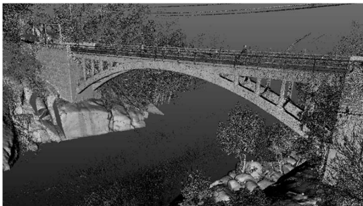
Figure 6. Point cloud after the optimization
