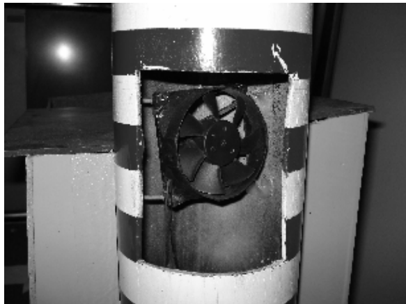
Figure 4. Fan inside the chimney
