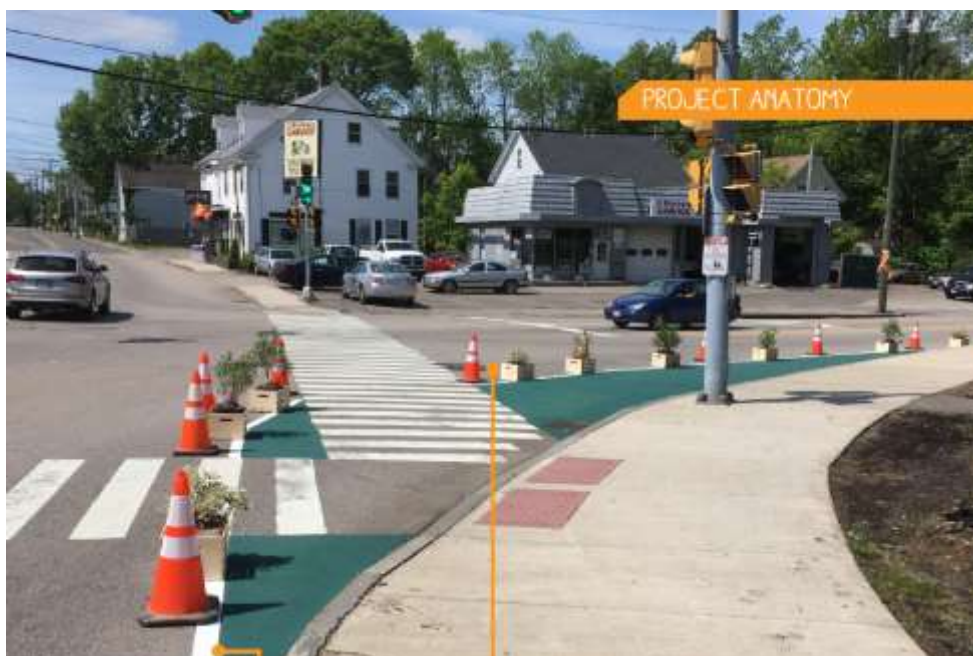
Figure 15: Curb extension in Portsmouth, USA (Source: Lydon, 2016)
