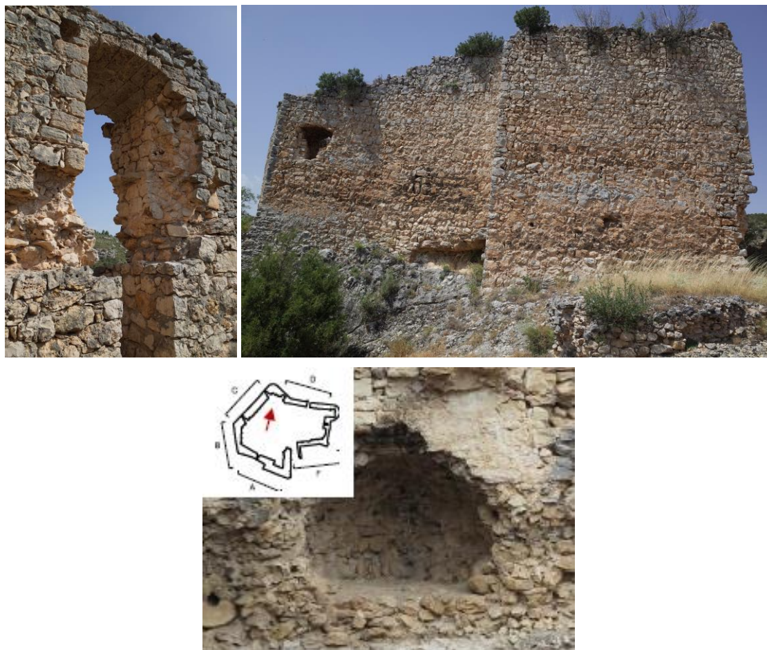
Figure 12:Castle in the state of degradation due to abandonment
