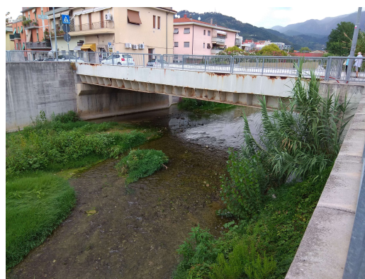
Figure 2. Bridge on “Via Gino Menconi”
