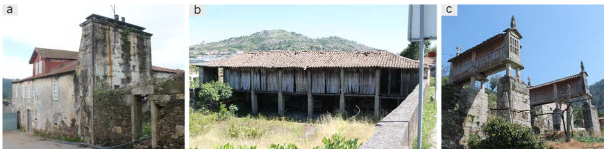
Figure 7 – (a) “fumeiro” chimney (Barcelos); (b) threshing floor and “varandão” (Braga); (c) two elevated “espigueiros” (Ponte da Barca).
