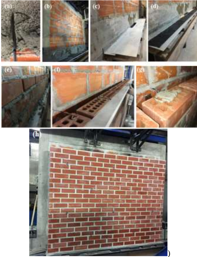
Figure 5. Construction phases of masonry specimens
