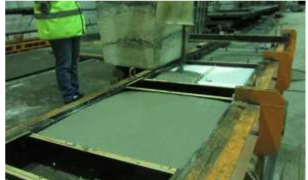
Figure 8 - Casting the top SFRSCC layer.
