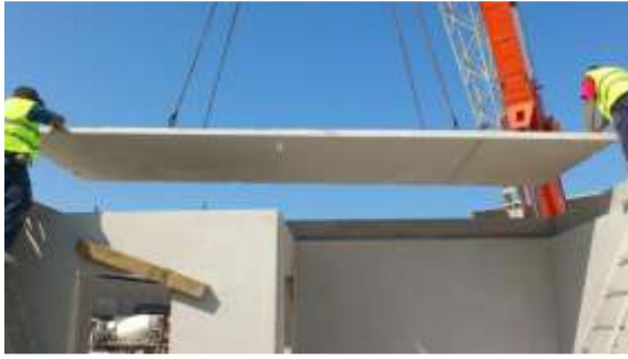
Figure 10 - Installation of the roof sandwich panels.
