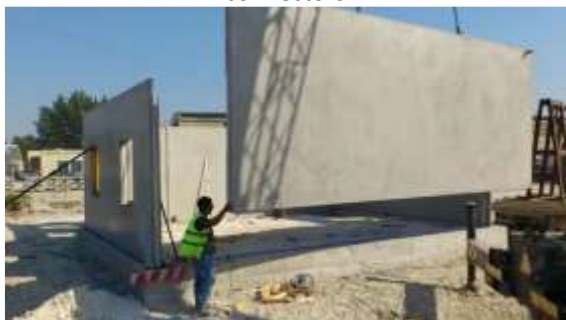
Figure 9 - Installation of the sandwich panels.
