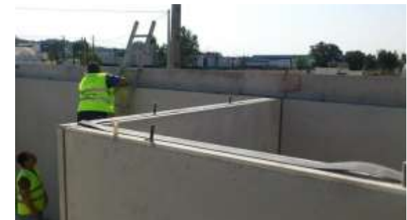
Figure 9 - Installation of the sandwich panels.
