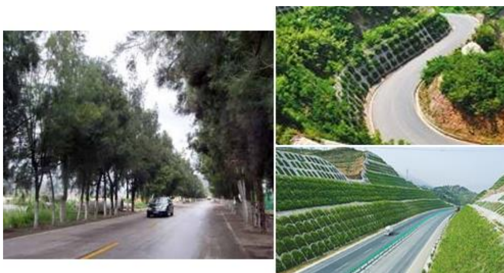
Figure 19 - Road shelter forest and slope protection
