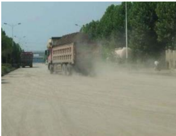
Figure 1 - Dust pollution from road construction ( https://image.baidu.com/ )
