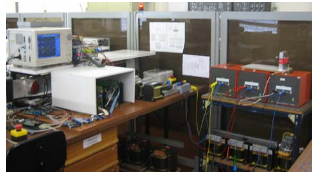
Fig. 2. Laboratory prototype of the Shunt Active Filter.
