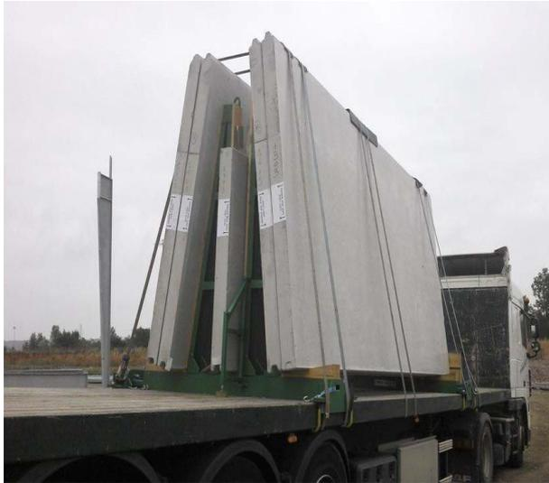
Figura 101: Processo de transporte de painéis de betão ([https://www.mekaglobal.com/content/images/uploads/1024x768/3\\_1952.jpg](https://www.mekaglobal.com/content/images/uploads/1024x768/3_1952.jpg))
