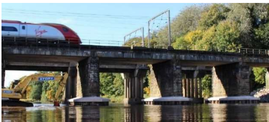
Figure 2. Eden Viaduct bridge. [32].
