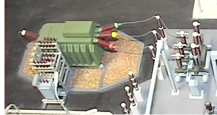
Figure 10. Close-up on main transformer (left) and circuit breakers (right)
