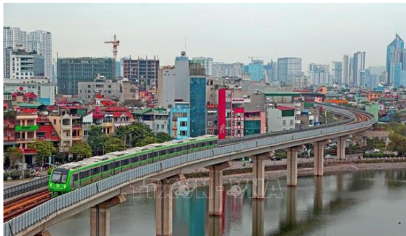
Fig. 3 – Cat Linh-Ha Dong railway bridge
