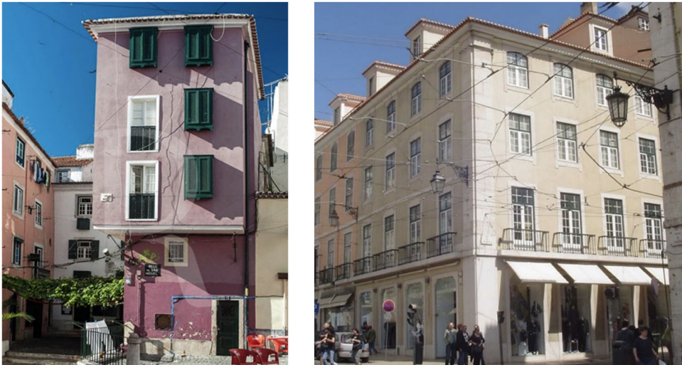
Figure 5. Unreinforced masonry buildings in the Lisbon Metropolitan Area: ‘Pre-Pombalino’ buildings (a) and ‘Pombalino’ buildings (b).
