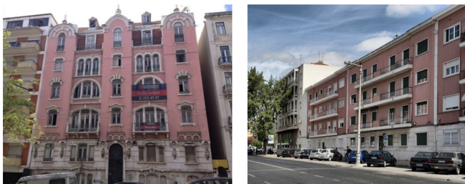
Figure 6. Unreinforced masonry buildings in the Lisbon Metropolitan Area: ‘Gaioleiro’ buildings (on the left) and ‘Placa’ buildings (on the right).
