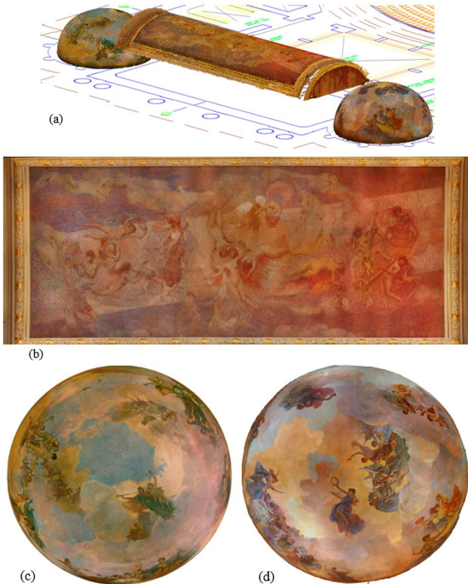
Figure 6 – Intrados of the domes and vault [60]: (a) point cloud; (b) orthophoto of the vault; (c) orthophoto of the dome of Av. Treze de Maio; (d) orthophoto of the dome of Av. Rio Branco. Images: Adolfo B. Ibáñez.
