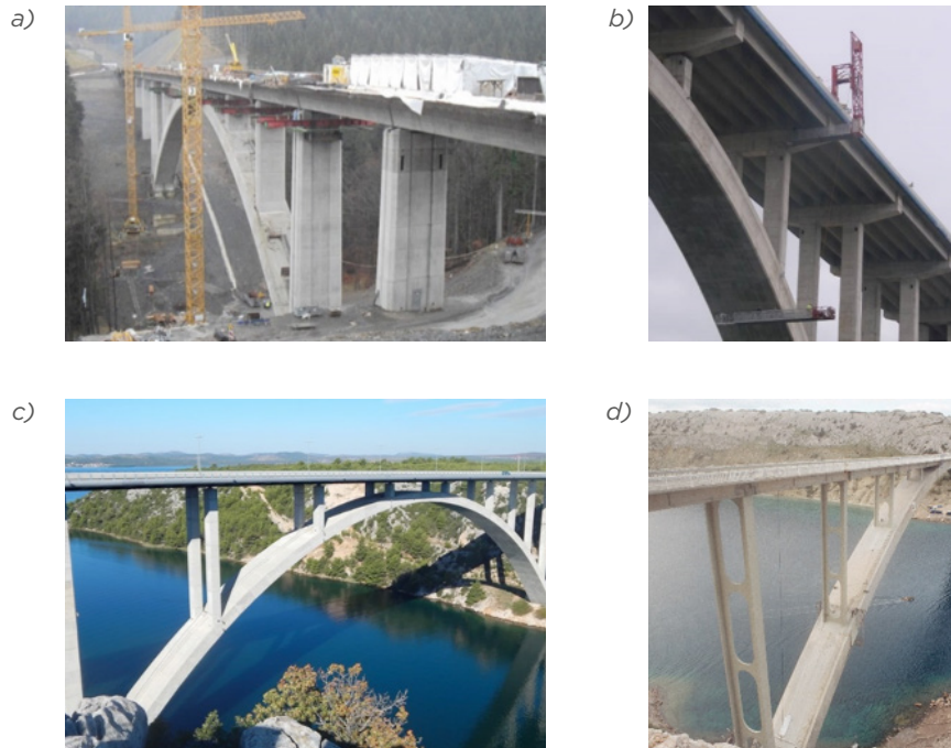
Figure 9.10 Pier types
