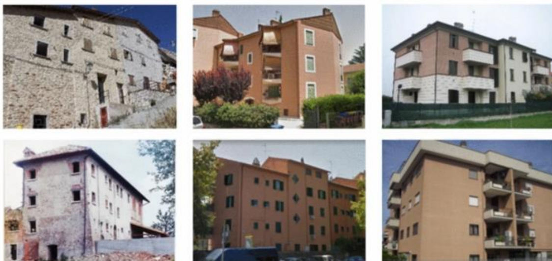
Figure 4.1 Typical 3- and 4-storey URM buildings of Italy [retrieved from (Donà et al. 2020)].
