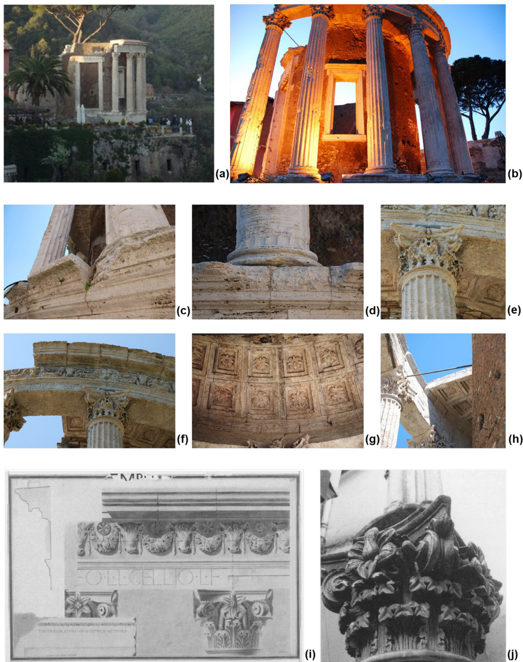
Fig. 2. The Vesta Temple in Tivoli. Upper: (a) view of the temple and the cliff, (b) global view. Middle: architectural details (c) podium, (d) column without plinth, (e) capital, (f) entablature, (g) coffered ceiling, (h) cella in irregular opus reticulatum . Bottom: reconstruction of architectural details (i) Royal Academy lecture's drawing of the entablature by Sir John Soane at Sir John Soane Museum with the reconstruction of the frieze's decoration, (j) full-size replica of the capital at Sir John Soane's Museum [43].
