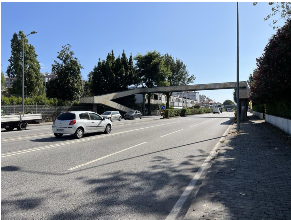
Figure 41: Current state of João Paulo II Avenue (own author)
