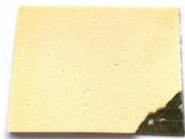
Figure 2.10. Cut-out piece of the PUR foam infilled CFS profile with delamination between the foam and the steel [76].
