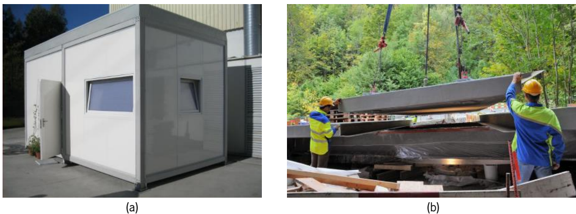
Figure 2.2. Current and potential applications of composite sandwich panels: (a) temporary shelter [18]; (b) bridge decks [20].
