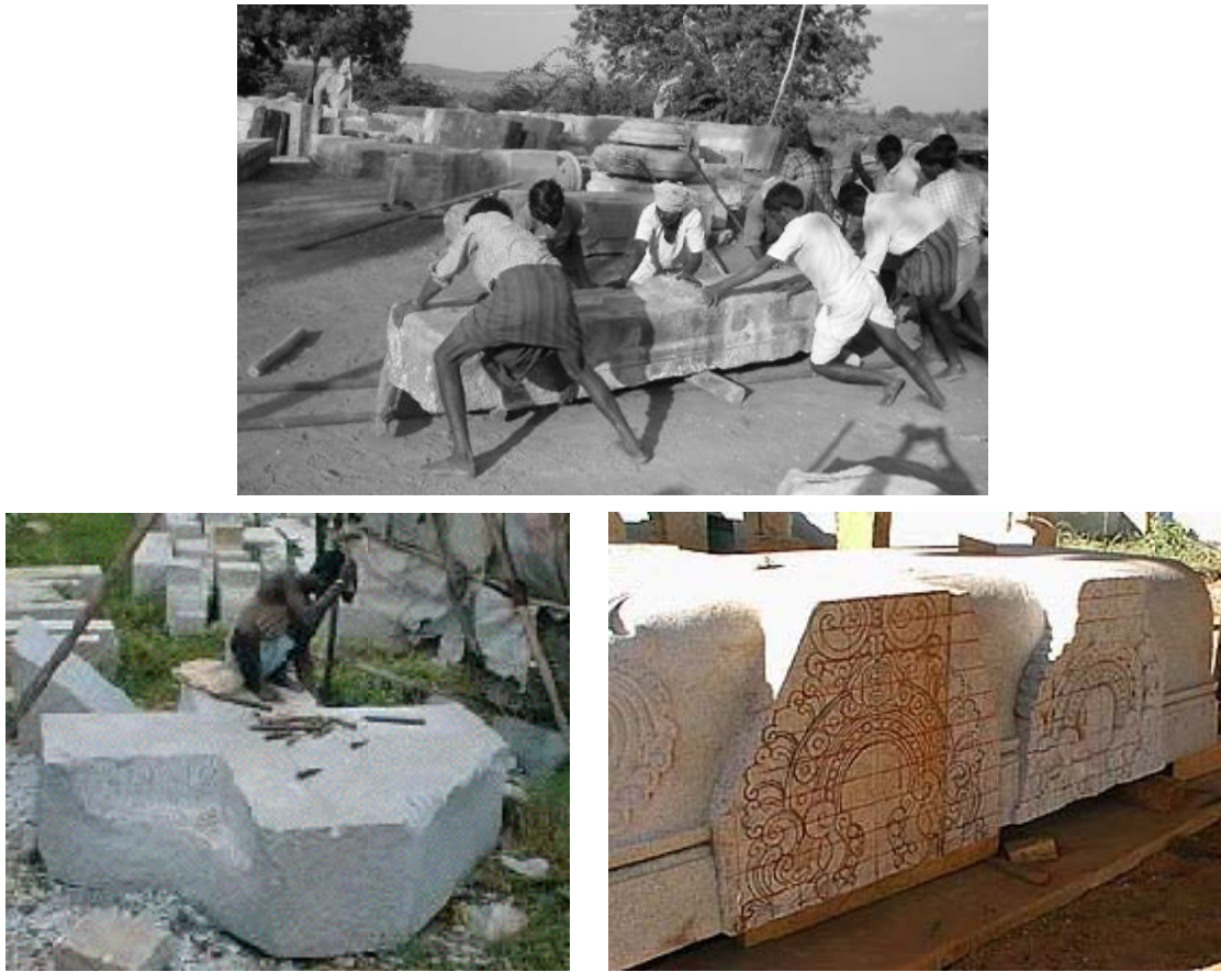
Figure 6: Transportation and carving of stones
