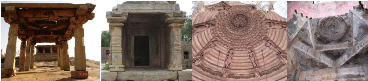
Figure 4: Trabeated system and the internal ceilings of the Hindu temple
