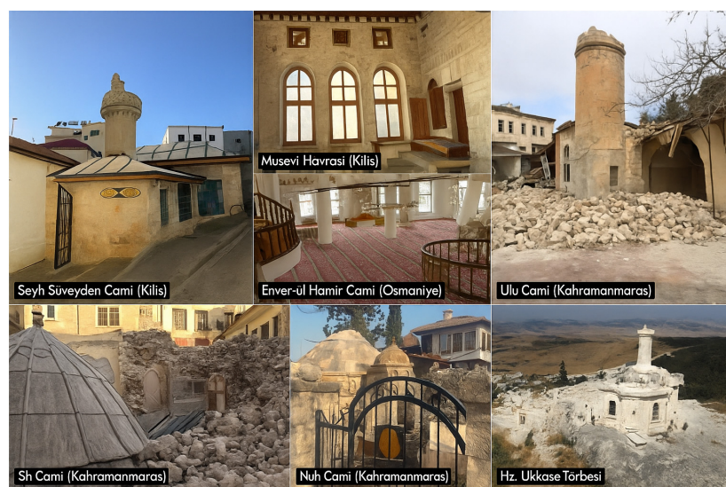
Figure 5. Examples of historical buildings damaged or destroyed in the 11 provinces impacted by the 6 February 2023 Kahramanmaraş earthquakes [8].
