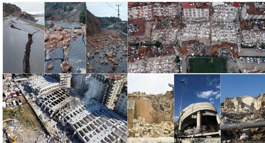
Figure 4. Examples of the widespread destruction caused by the 2023 earthquakes in the region, including surface ruptures, landslides, and the collapse of residential, historical, and public buildings [7].
