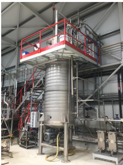
Figure 7 - Industrial fermenter with an operational volume of 5000 L located in AlgaFarm facilities.
