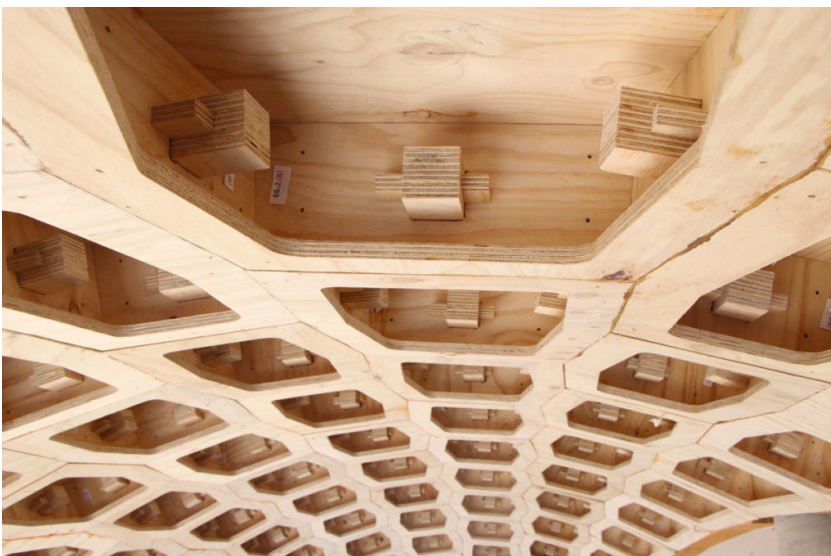
Wood-only connectors inspired by handcrafted carpentry and cabinet-making
