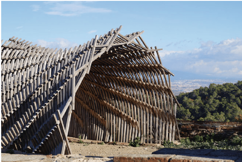
Figura 8.1.15. Vista geral do Pavilhão. Fonte: https://cargocollective.com/andreaquartara/filter/triangulation/Fusta-Robotica-Pavilion
