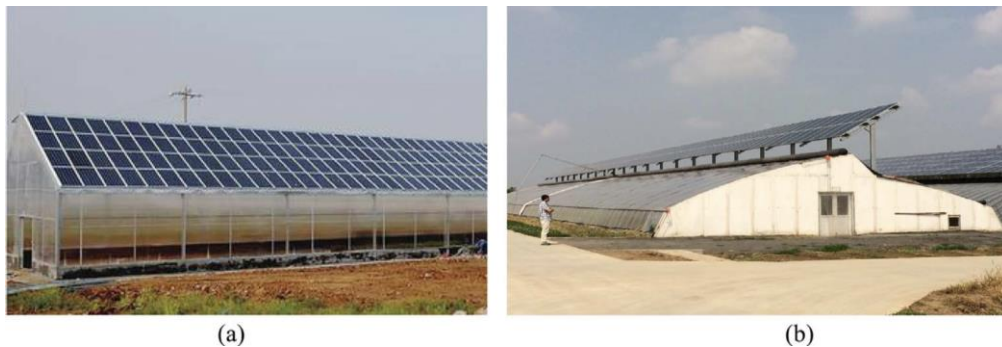
Figure 12 - Two possible ways to place opaque solar panels on greenhouses, taken from [15]
