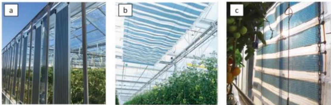
Figure 18 - Different ways of installing Organic STPV modules in a greenhouse facing different directions. Adapted from ([8])
