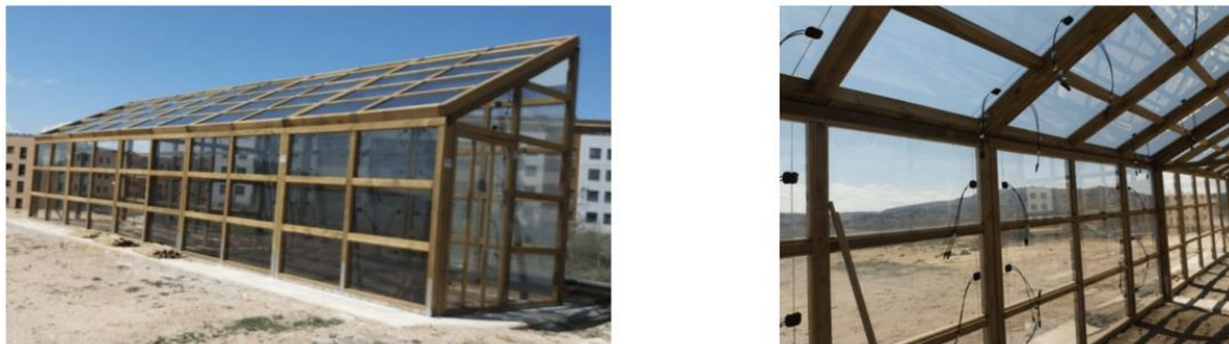
Figure 16 - Greenhouse setup used for the study [21]
