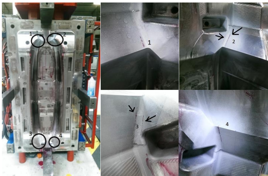
Figure 265 – Images of the locations where fatigue cracks appeared in the tool.
