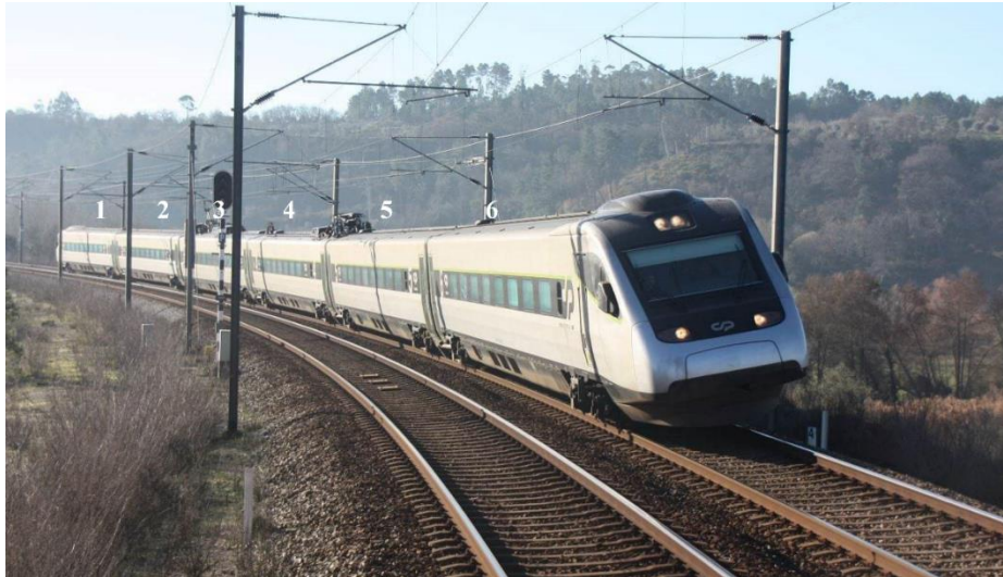
Figure 5.3. CPA 4000 series train in operation.
