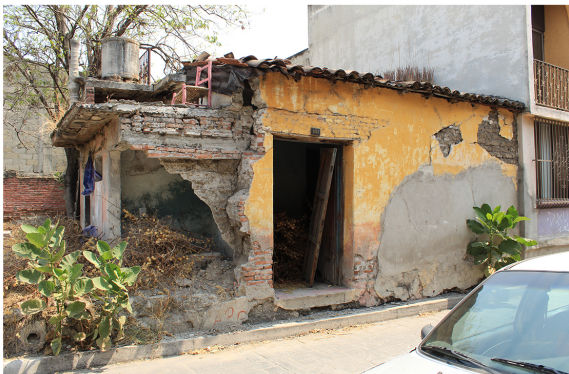
Grade 3: Substantial to heavy damage (moderate structural damage, heavy non-structural damage).
