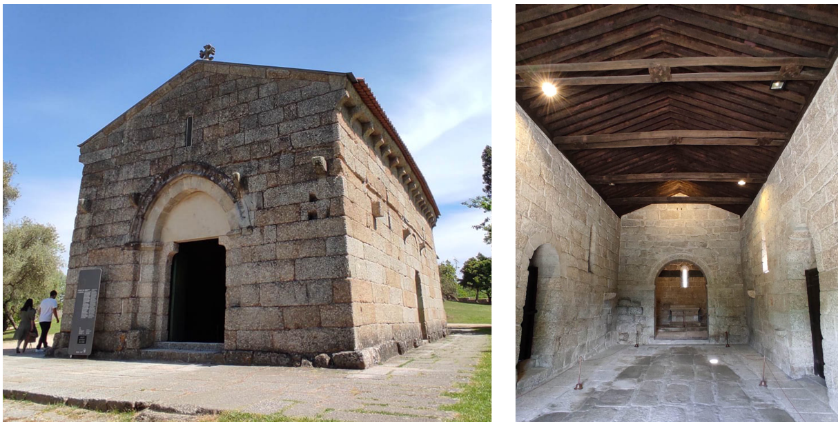
Figure 3.8: Church of São Miguel, Guimarães, Portugal: main façade (a) and nave view (b).
