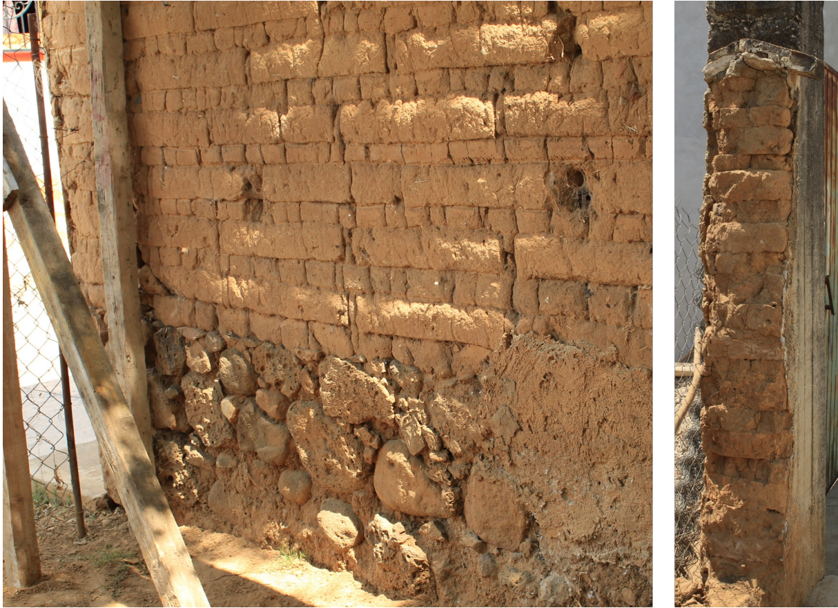
Figure 7.6: Typical adobe configuration in a house in the municipality of Tlayacapan.
