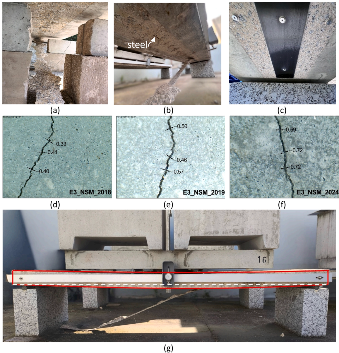
Fig. 9. Monitoring of time-dependent responses in CFRP-strengthened slabs: concrete cohesive-dominated failure modes observed in (a) E3 and (b) E5; (c) soffit of slab with EBR-GA system in E4 after six years of exposure; crack widths (in mm) measured for NSM slab after (d) one, (e) two, and (f) six years of exposure in E3; and (g) deflected shape of the EBR-GA system in E5 after six years of exposure.
